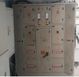
Currently, there is a down time of around 10 mins, when an operator manually switches from grid power (during power failure) to source the power from diesel generator. Operator has to disconnect the line from Solar panels, as the power from diesel generators is expected to interfere with the solar panels. Diesel generator is then started and is connected to load.
